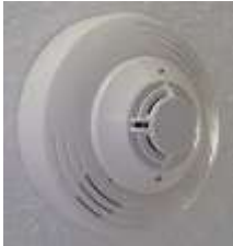
Smoke and Heat Detector Button for silencing the Smoke & Heat Detector (on the wall)
