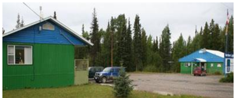
Figure 9 Dease Lake Access Centre
