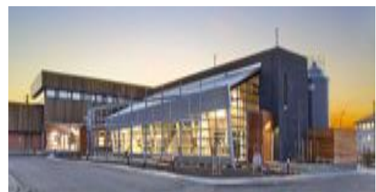
Figure 2 Energy House, Dawson Creek Campus
