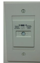
Smoke and Heat Detector Button for silencing the Smoke & Heat Detector (on the wall)
