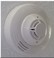
Smoke and Heat Detector Button for silencing the Smoke & Heat Detector (on the wall)
